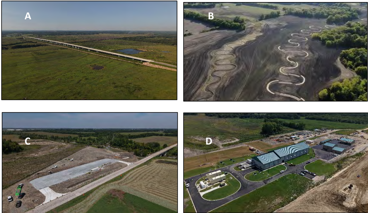
Figure 2. Lake Ralph Hall improvements underway. A) SR 34 Bridge; B) Stream mitigation downstream of Leon Hurse Dam; C) Ladonia Fossil Park; D) Lake Ralph Hall Pump Station and Maintenance Facility
